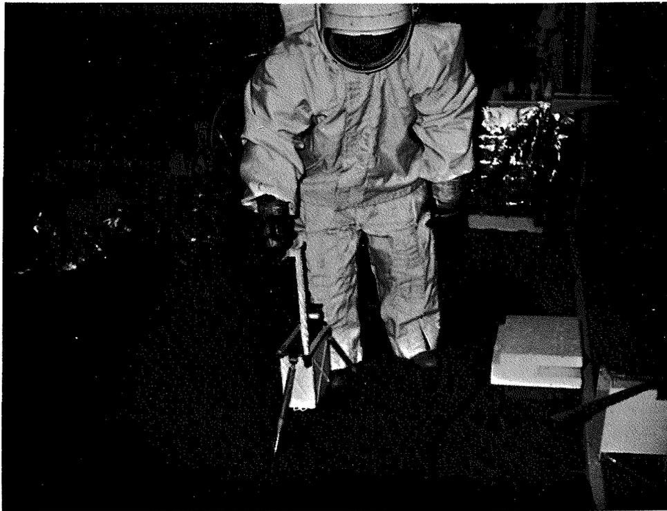
FIGURE #5 Use of EHT shank as gnomon for orientation of CPLEE to E-W axis.
